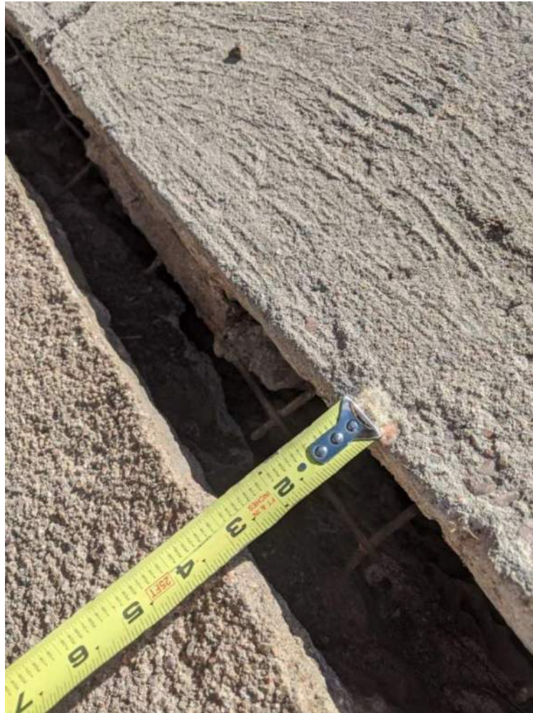
12: I25 bridge, the concrete slabs from photo 11 have separated and will need to be stabilized if Greenway will go near them or below them
