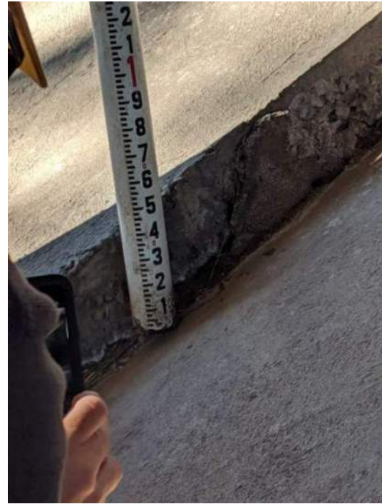
8: I25 bridge, existing slope paving has heaved (north side)
