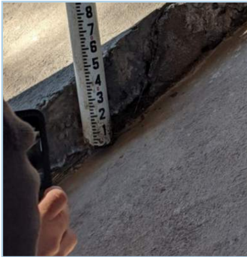
I-25 BRIDGES, SLOPE PAVING HEAVED
