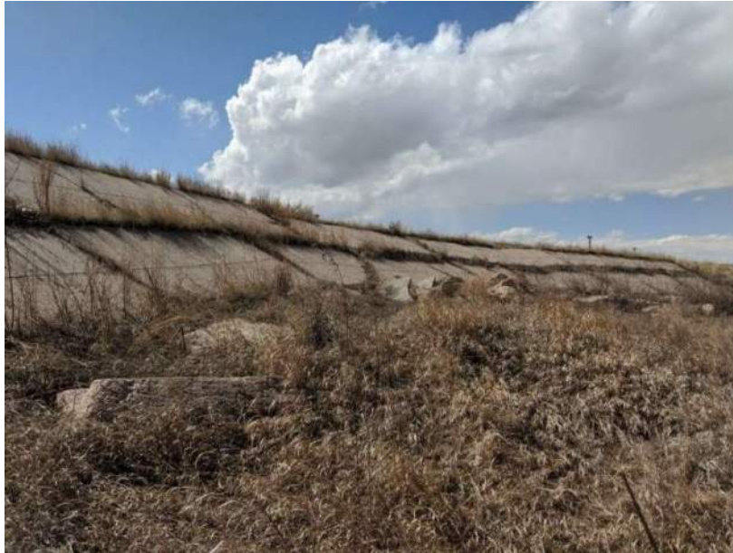
11: I25 bridge, standing under bridge, south bank, looking west: south west bank is armored with concrete slabs and riprap
