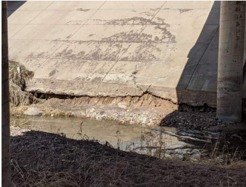
9: I25 bridge, scour at slope paving (north side)
