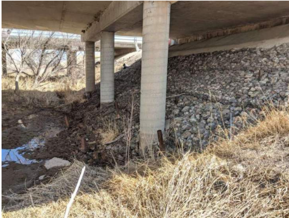
10: I25 bridge, south side has gabion basket slope protection under the bridge (not concrete slope paving)
