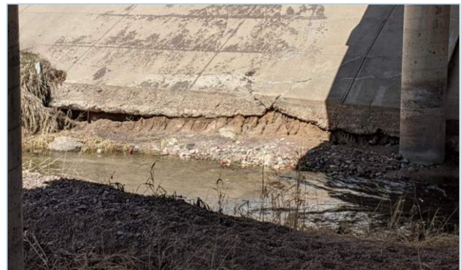
SCOUR AT NORTH BANK SLOPE PAVING
