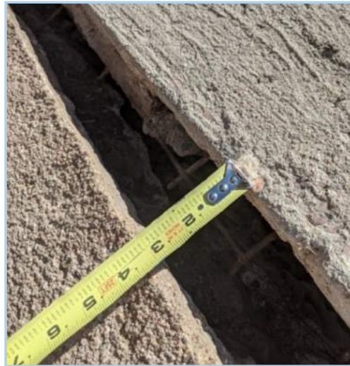
I-25 BRIDGES, SLOPE PAVING SLABS SEPARATING
