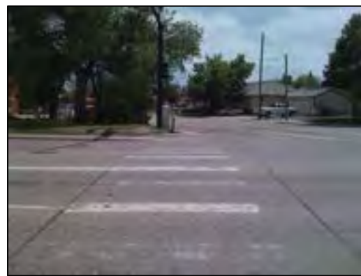
Figure 9. Faded crosswalks can be hazardous to pedestrians
