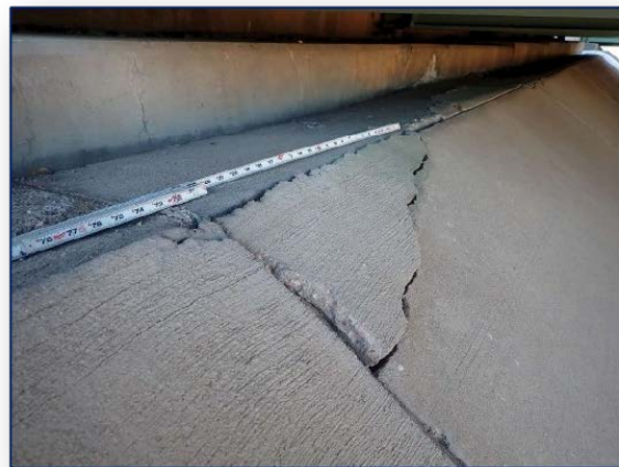
Figure 13b - I-80 Bridge Structure
