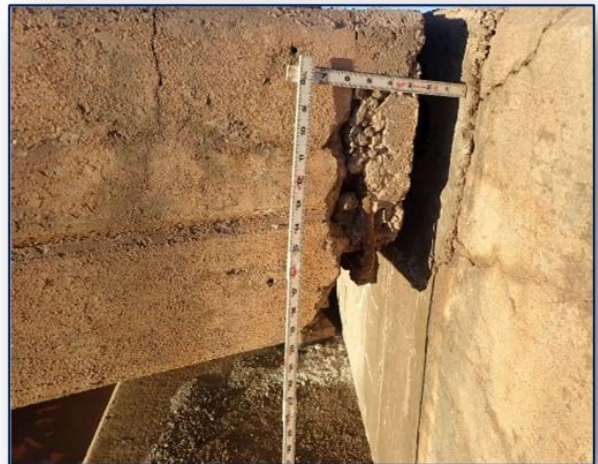
Figure 13a - I-80 Bridge Structure
