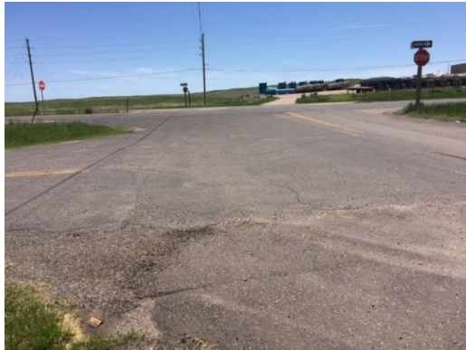
Figure 2.4 High Plains west of U.S. 85/ South Greeley Highway Looking east
