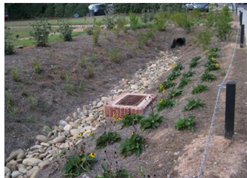
Figure 5.4 Linear / Conventional Detention
