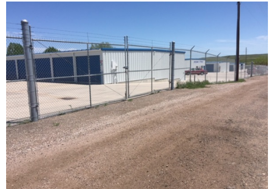
Figure 2.5 High Plains Road at Speedway Storage looking northeast
