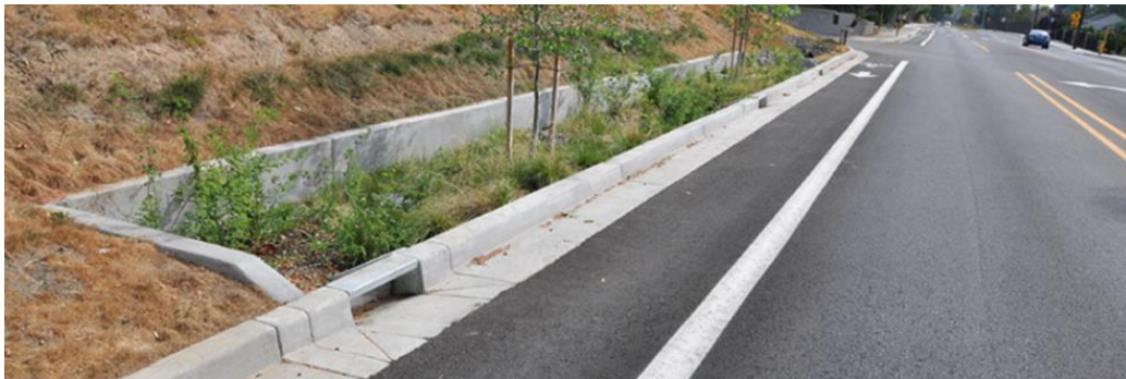
Figure 5.5 Gutter Turnouts
