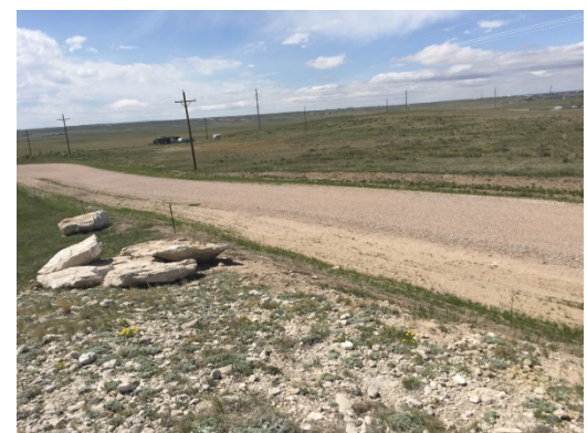
Figure 2.7 High Plains Road at west cul-de-sac looking west
