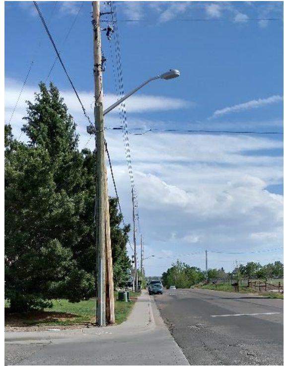
Photo 3 Double utility poles found within project corridor
