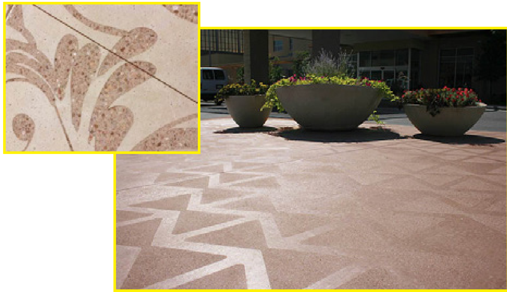
CONCRETE SANDBLASTING
