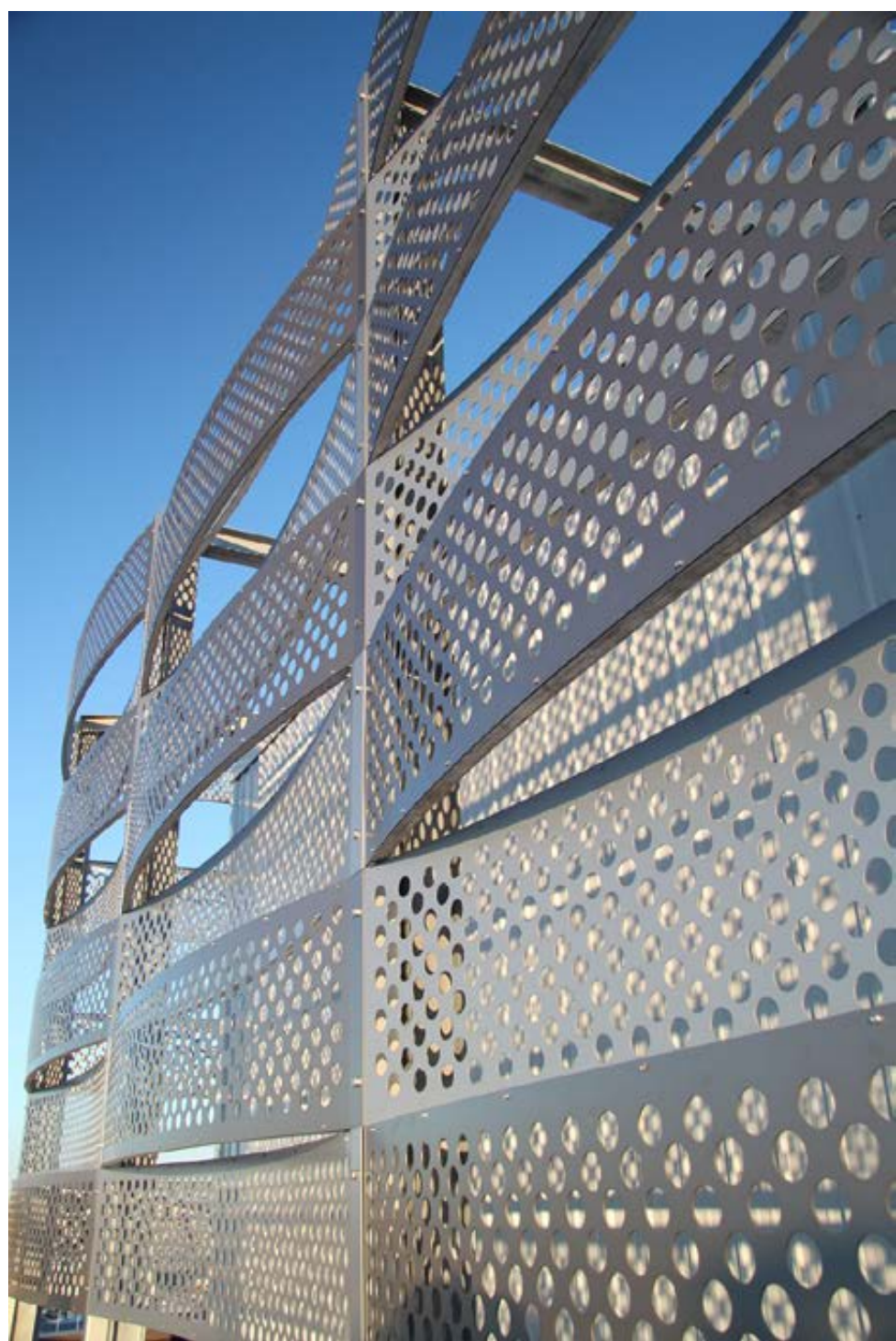
B) Perforated Metal Cladding Screens
