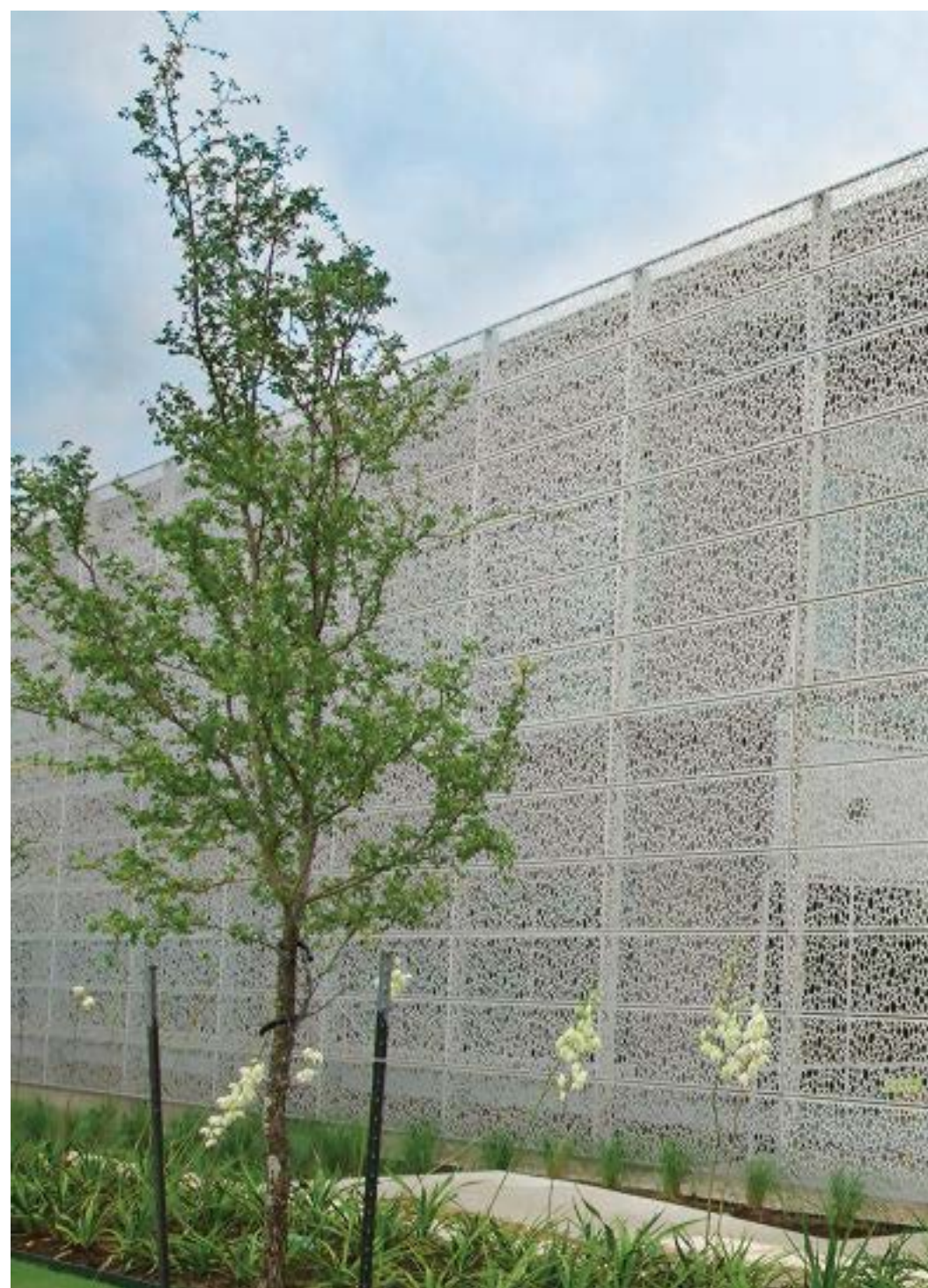
B) Perforated Metal Cladding Screens
