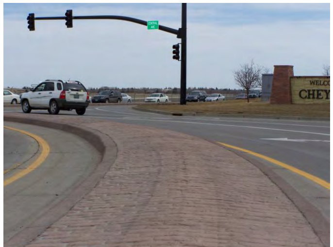
Central Avenue Median using Stamped Concrete and Monolithic Concrete Coloring Additive Texturing and Coloring Option B
