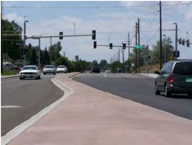
12 th Street (Left) and Vandehei Interchange (Right) Median using Monolithic Concrete Coloring Additive with Alternating Broom Finish
