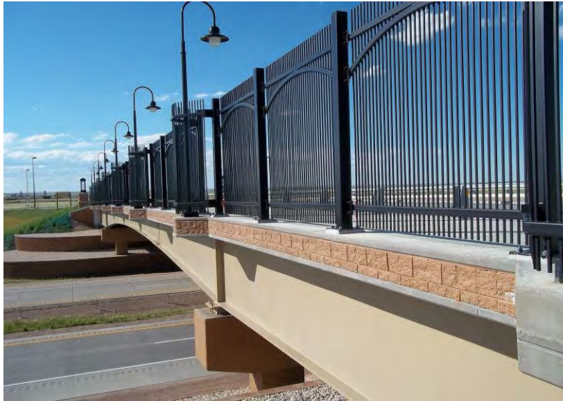
I-25 High Plains Interchange Pedestrian Fence Detail Option C
