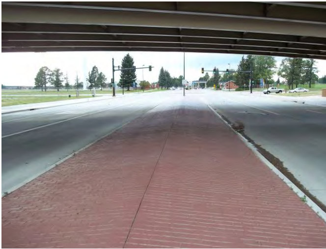
West Pershing Blvd. (Left) and High Plains Interchange (Right) Median using Stamped Concrete and Penetrating Stain Coloring Agent
