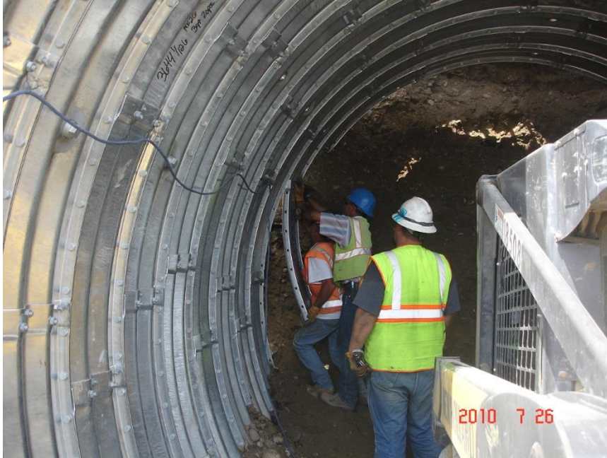
Figure 13: Alkali Creek Tunnel - Liner Plate Assembly
