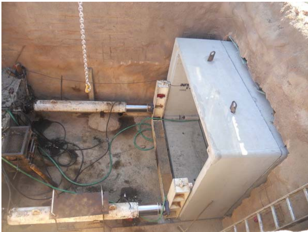
Figure 10: Image of Box Culvert Jacking
