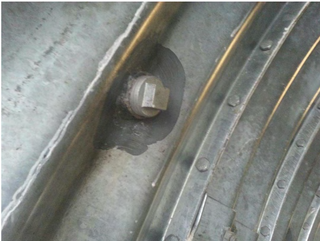
Alkali Creek Tunnel, Grout Holes
