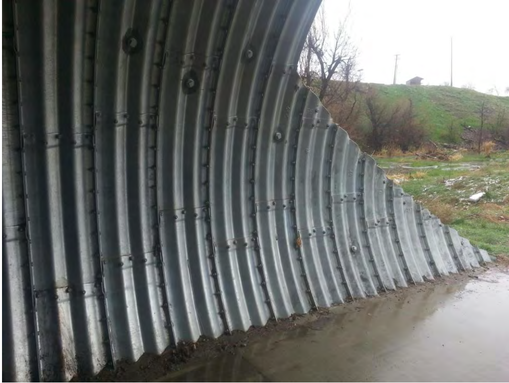
Alkali Creek Tunnel, Steel Plate Pipe
