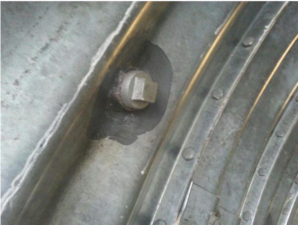
Alkali Creek Tunnel, Grout Holes
