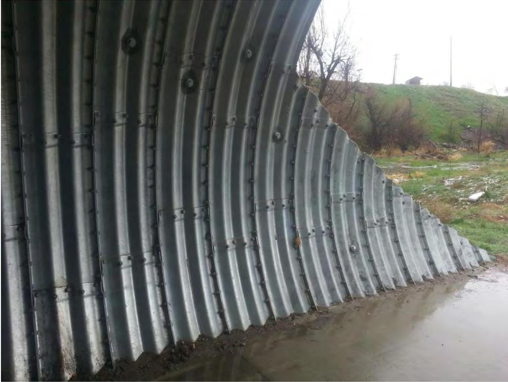
Alkali Creek Tunnel, Steel Plate Pipe
