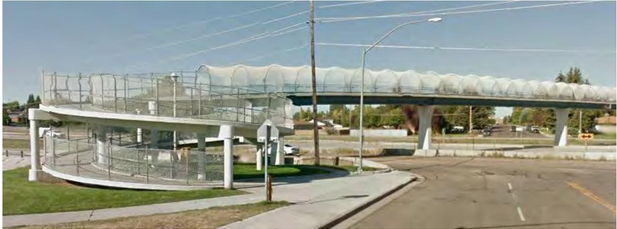
2. The ramp at the south side of Option B is located between Campstool Way and Campstool Road. There is quite a bit of land there, which allows for a switchback type ramp and possibly the use of import fill for a ramp rather than a structure. A consideration is sight distance for vehicles at the intersection. Another advantage of this location is that greenway users are brought to an existing intersection with a traffic signal. The existing signal could be modified to have pedestrian facilities.
