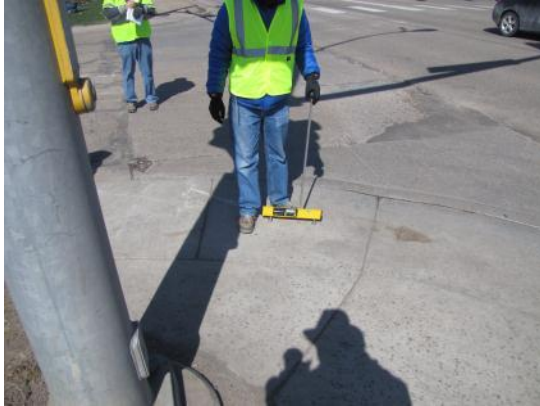
Exhibit 35 Slope of Pedestrian Ramp in SW Corner
