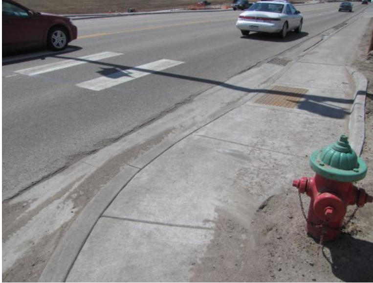
Exhibit 85 Fire Hydrant Limiting Clear Sidewalk Width
