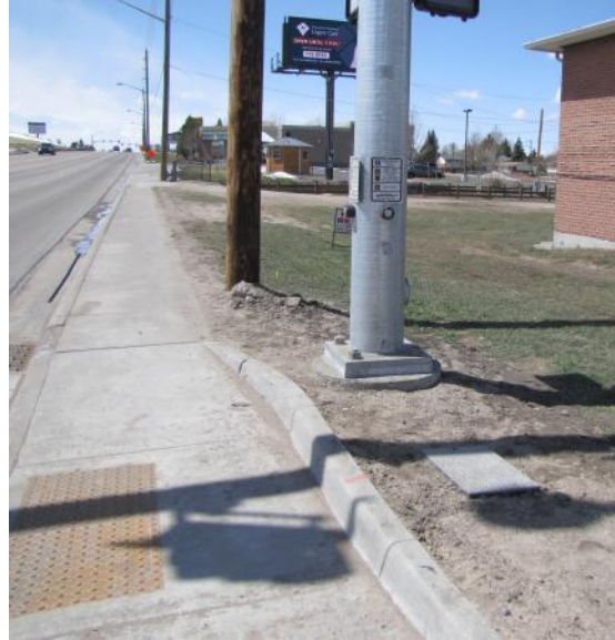
Exhibit 84 Inaccessible Pedestrian Push Button in NW Corner – Looking West
