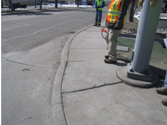
Exhibit 31 Sidewalk Width Near Signal Pole is 3'-6"
