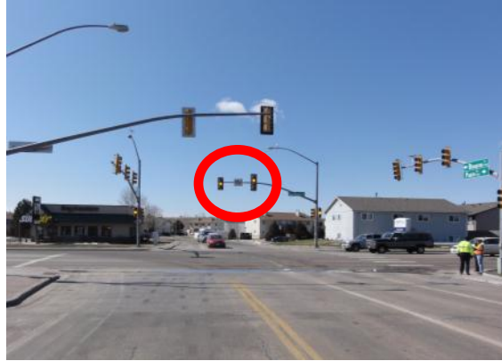
Exhibit 46 Southbound Approach – Channelization Sign between Signal Heads
