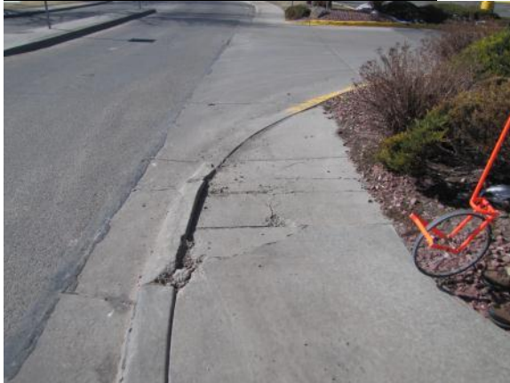
Exhibit 20 Cracked Sidewalk in SW Corner Looking South
