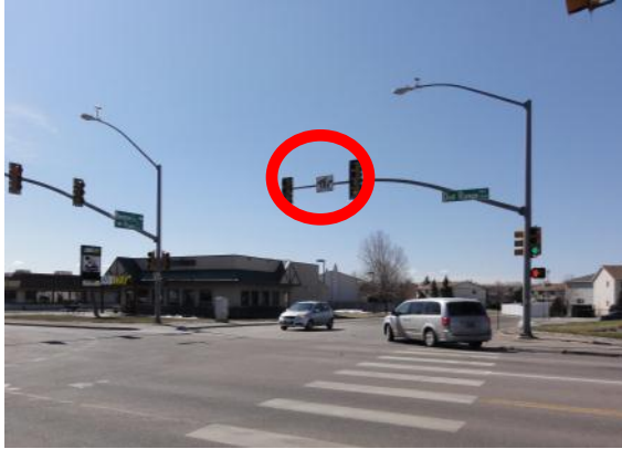
Exhibit 45 Southbound Approach – Channelization Sign between Signal Heads
