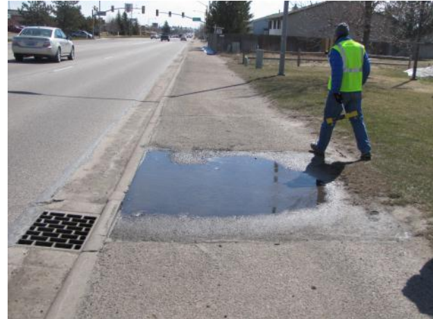
Exhibit 44 Water Ponding on Sidewalk
