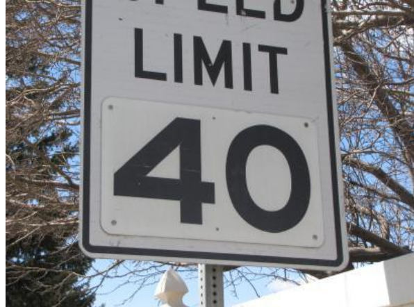
Exhibit 93 Panel to change speed limit
