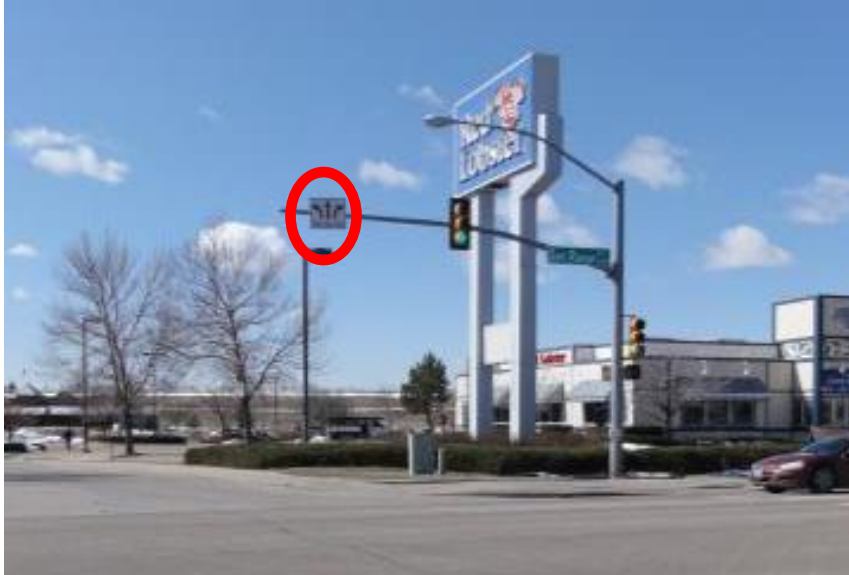
Exhibit 56 Low Reflectivity of Channelization Sign Mounted to Mast Arm Signal Pole
