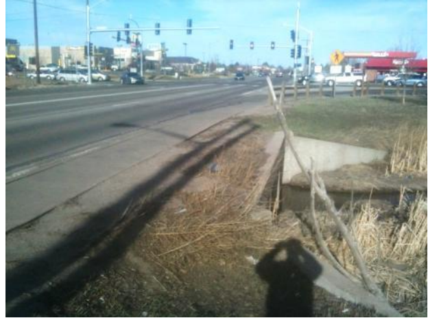
Exhibit 96 South Side Box Culvert
