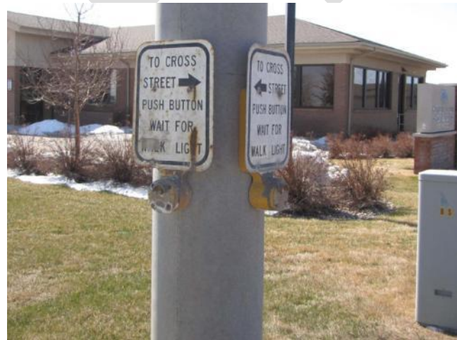
Exhibit 9 Example of Pedestrian Push Button and Sign
