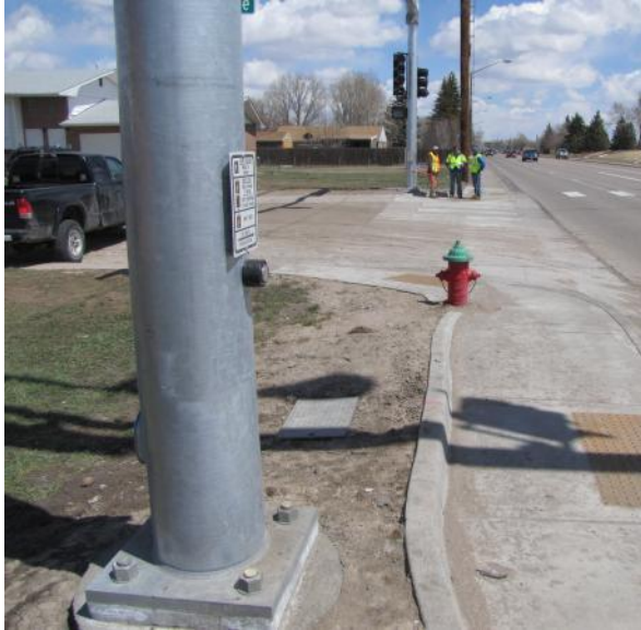
Exhibit 83 Inaccessible Pedestrian Push Button in NW Corner – Looking East
