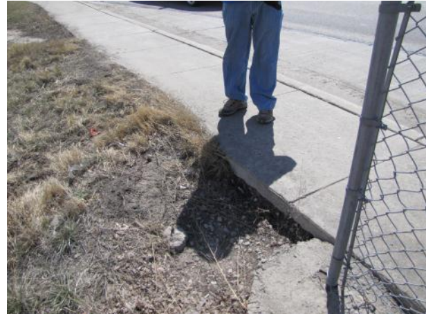
Exhibit 69 North side – sidewalk drop-off at box culvert – east of culvert
