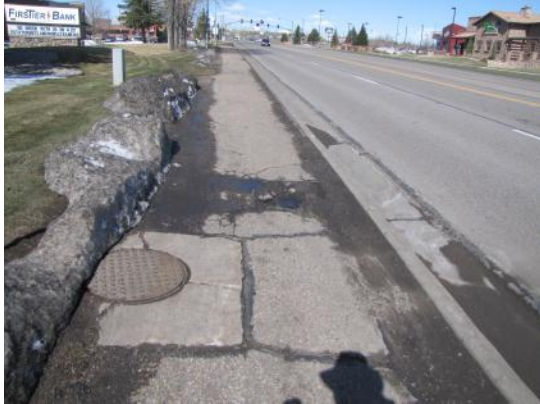
Exhibit 22 Cracked Asphalt Sidewalk – South Side
