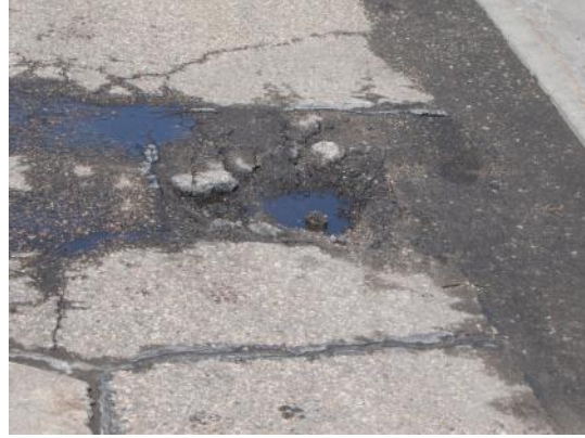
Exhibit 23 Pot Hole in Asphalt Sidewalk
