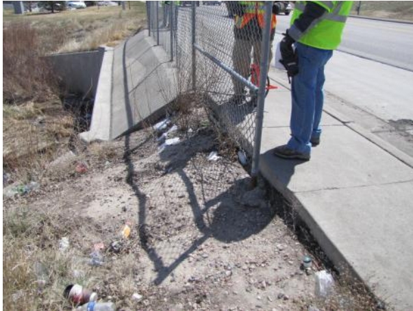
Exhibit 68 North side – sidewalk drop-off at box culvert – west of culvert
