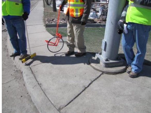
Exhibit 32 Sidewalk Width Near Signal Pole is 3'-6"
