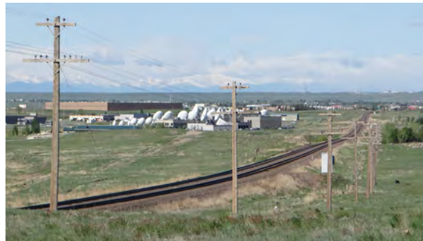
The future bridge will span these two main line railroad tracks.
