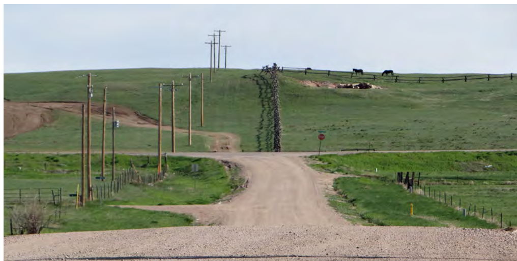
Looking north from the UPRR ROW, the photo shows the dirt road that will be rebuilt and then continue past E. Pershing up the hill toward US 30.
