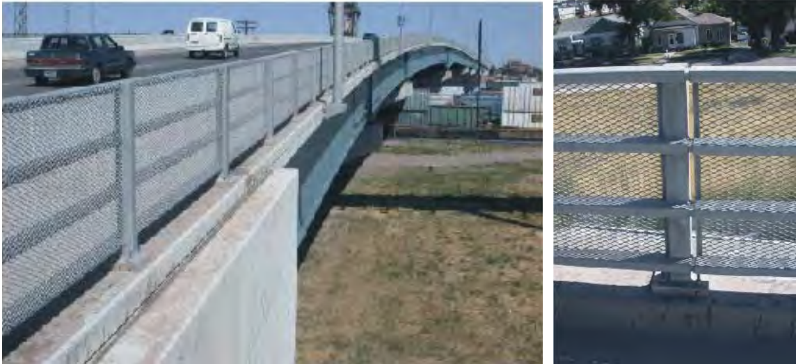
Figure 2. Existing Bridge Rail
