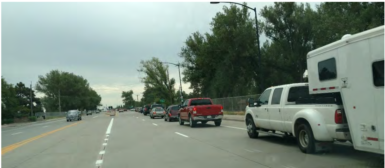
Figure 23: Eastbound Central Ave., west of Kennedy Road
