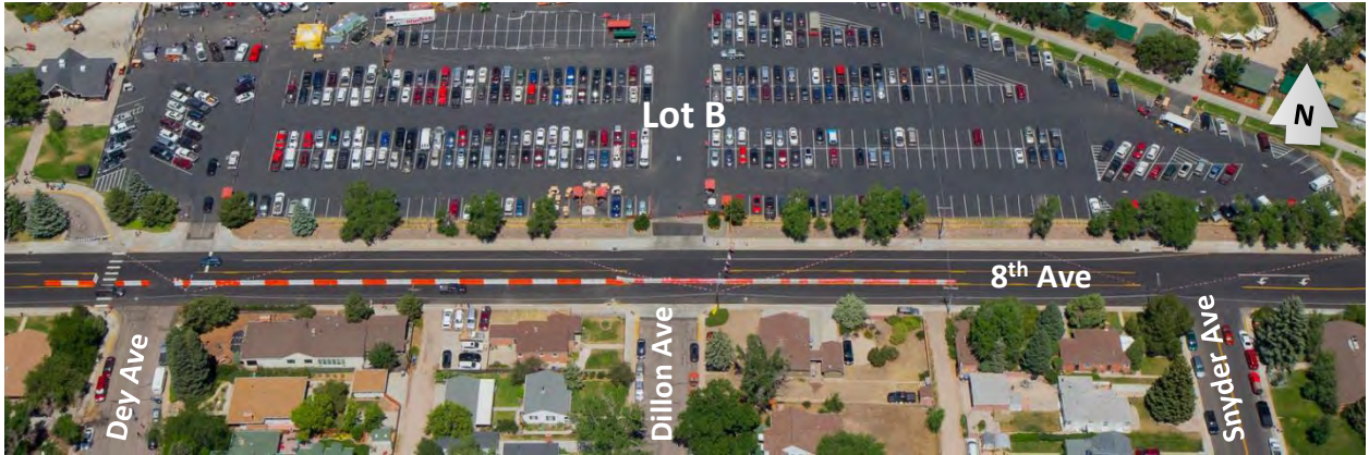
Figure 13: 8th Ave. Traffic Barrier (Image from Friday, July 28, 12:30 p.m.)
