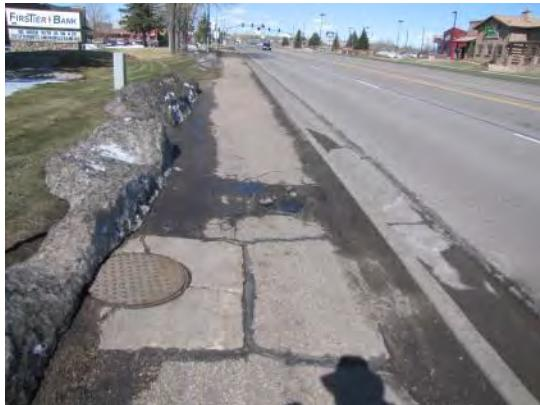
Exhibit 22    **Cracked Asphalt Sidewalk – South Side**
