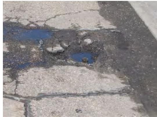
Exhibit 23    **Pot Hole in Asphalt Sidewalk**
