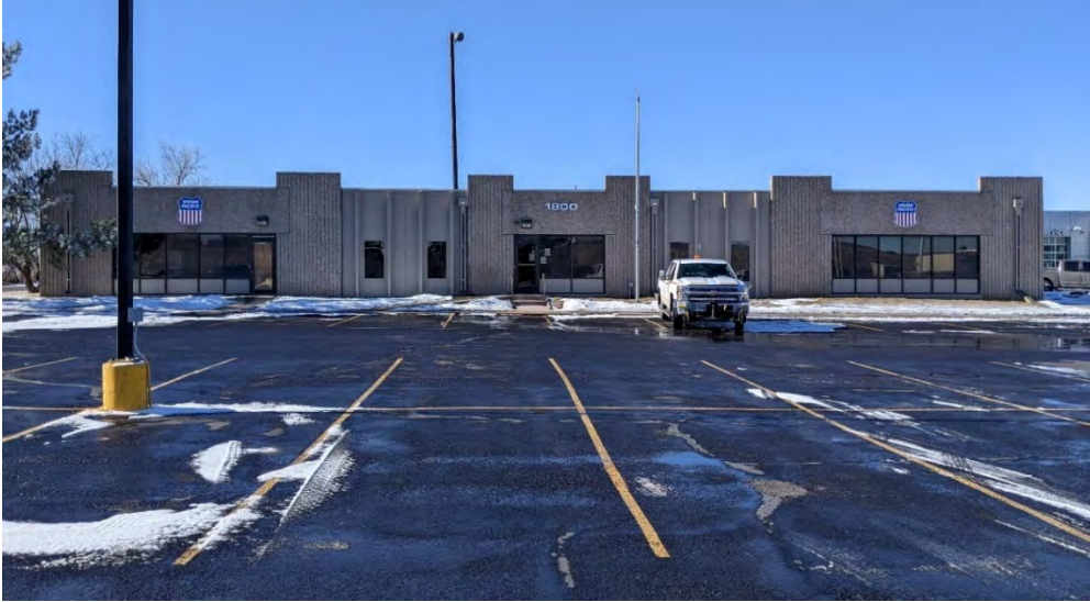
Figure 85: Future CTP Office
