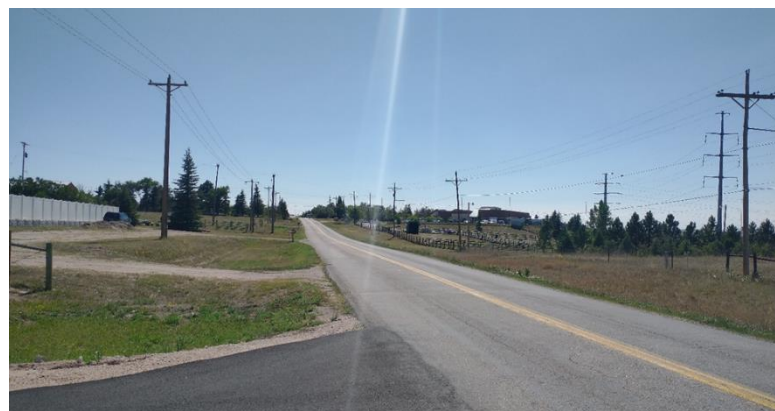
Figure 4 Utilities along the corridor
