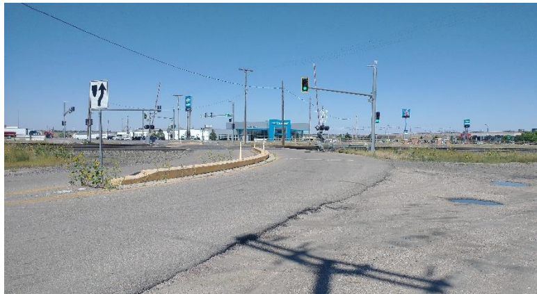
Figure 1 Southwest Drive intersection with Lincolnway
