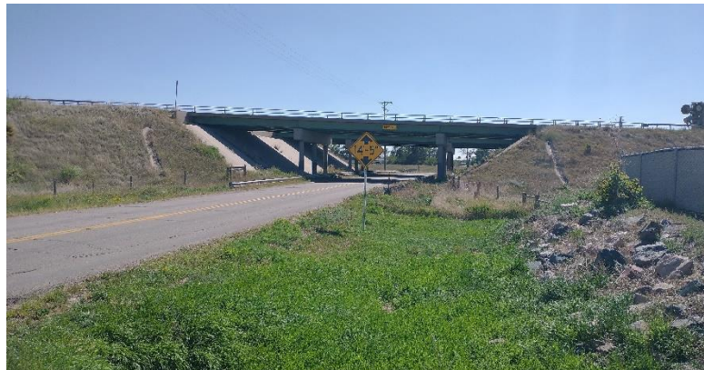
Figure 3 Narrow width under I-80 Bridge
