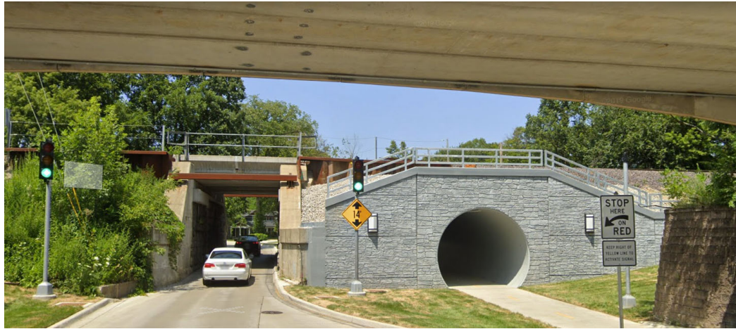
Taylor Avenue Underpass in Glen Ellyn, IL – UPRR
