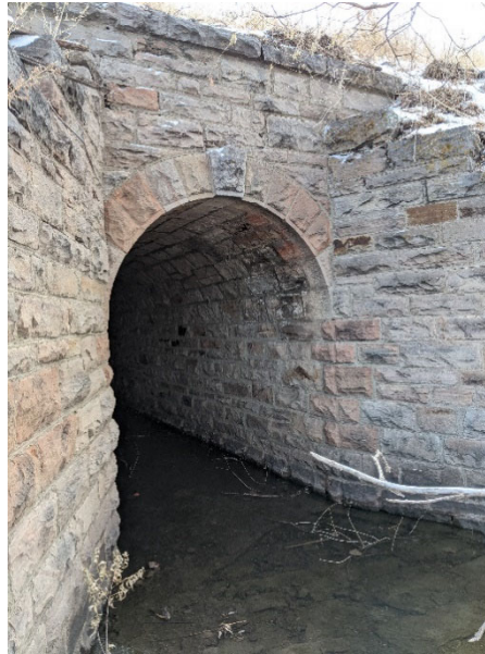
Existing historic Box Arch Masonry Structure
