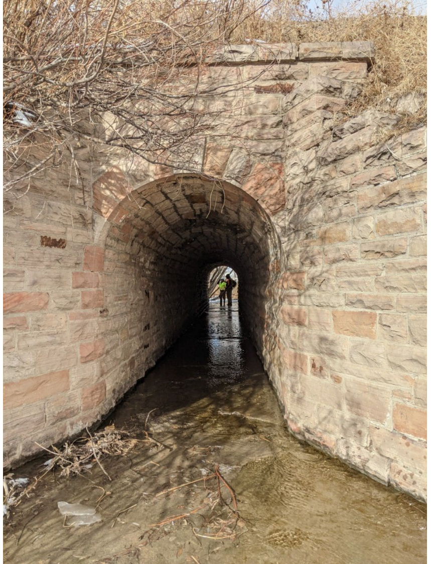
Figure 8: Masonry Arch Structure South Portal Looking North
