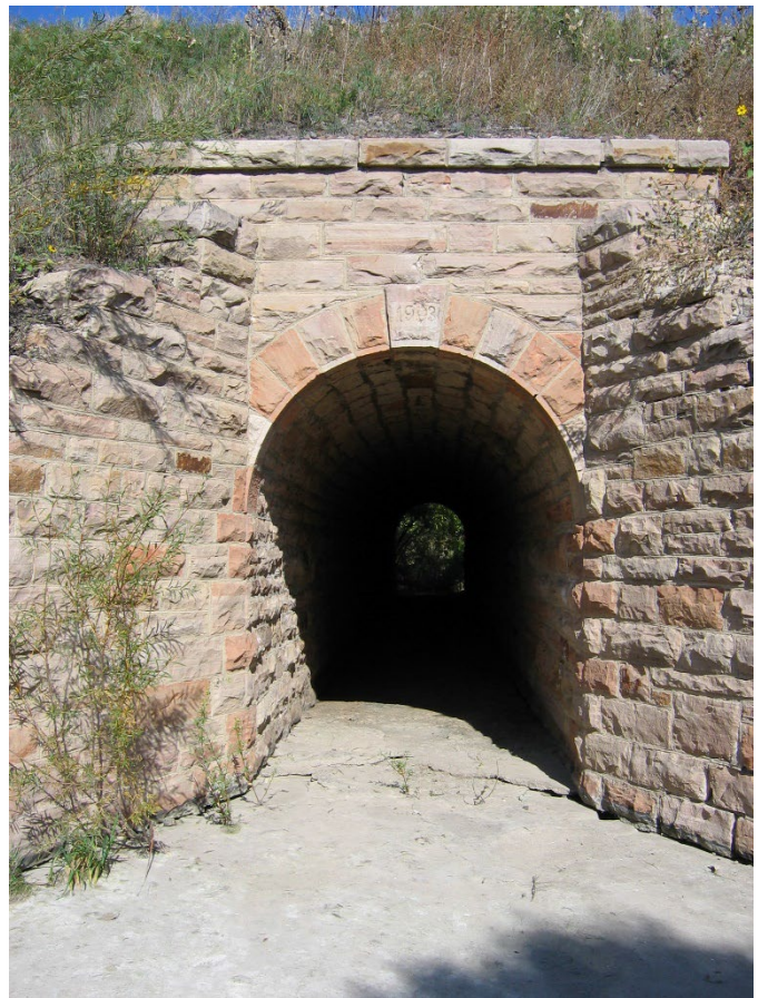
Figure 2: 1903 Structure constructed for Drainage Conveyance
