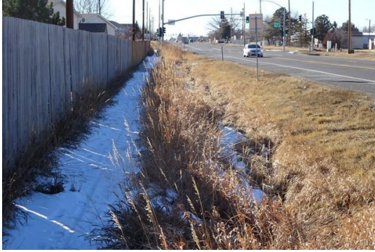
Drainage Ditch without Sidewalk
