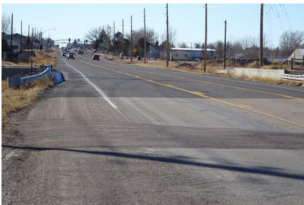
East Pershing at Dry Creek Culverts
