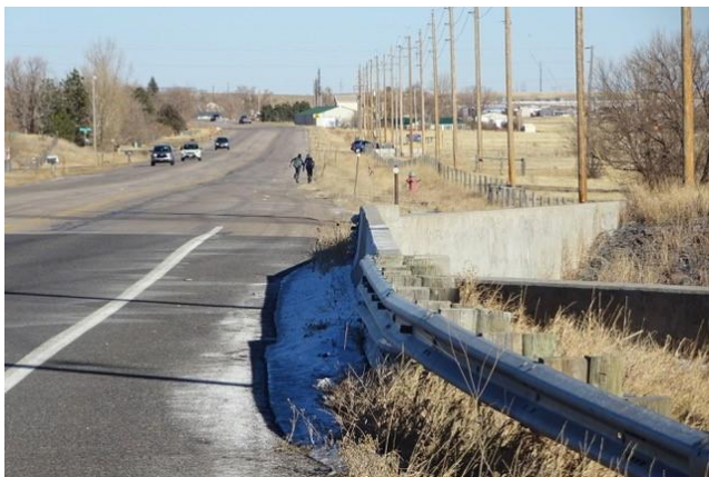
At the Dry Creek Culvers Looking East
