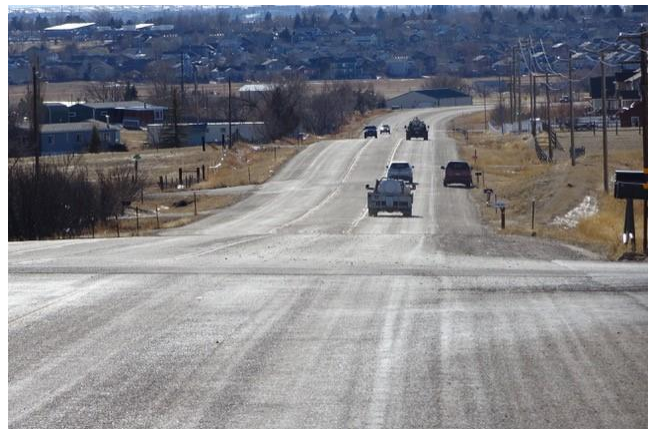
Eastern Section of Pershing Looking West
