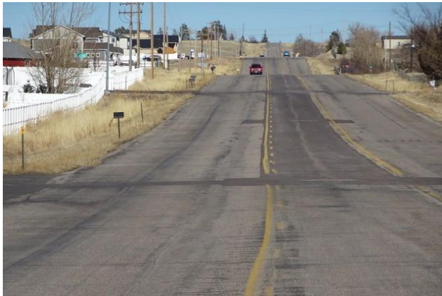
South of Saddle Ridge Looking East
