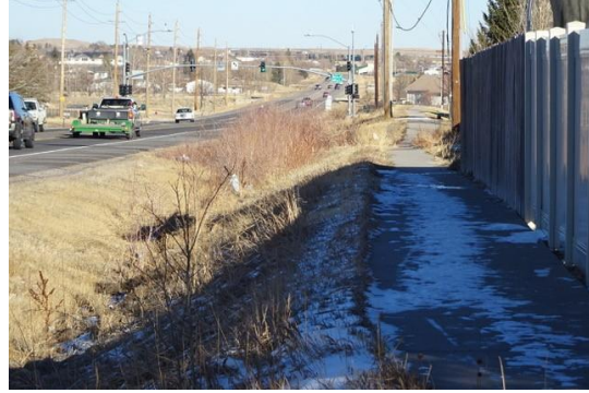
Drainage Ditch with Narrow Sidewalk
