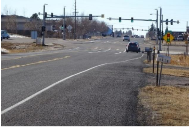
East of U.S. 30 Intersection Looking West
