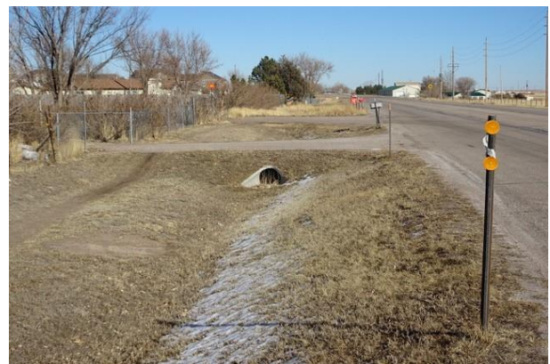
Pershing Drainage on the Northside
