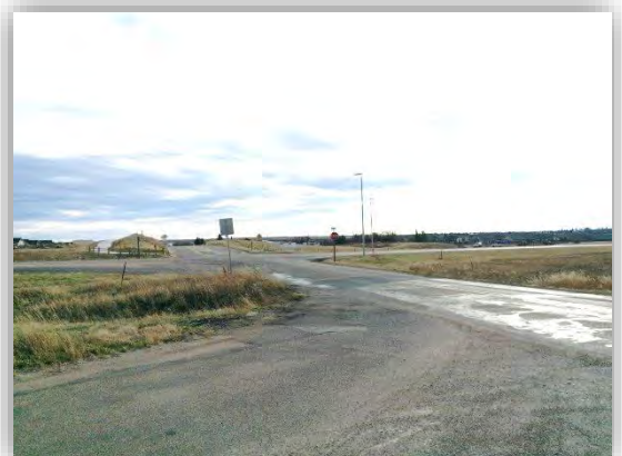
Figure 2.8 Whitney Road at US 30 (Looking southwest)
