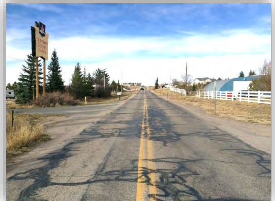
Figure 2.7 Whitney Road north of US 30 (Looking north)
