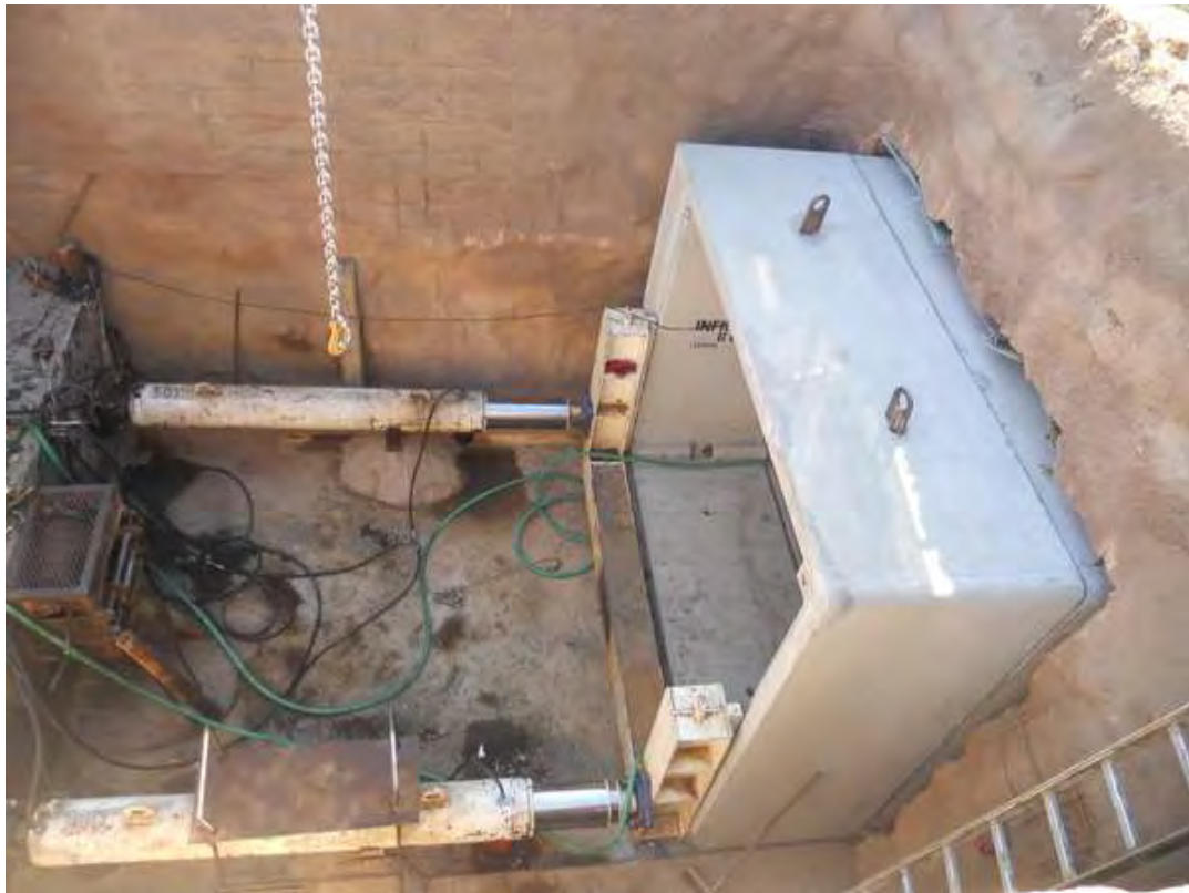
Figure 10: Image of Box Culvert Jacking
