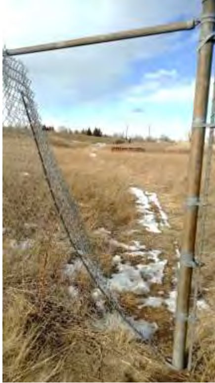
Figure 7: Hole in Chain Link Fence, looking north
