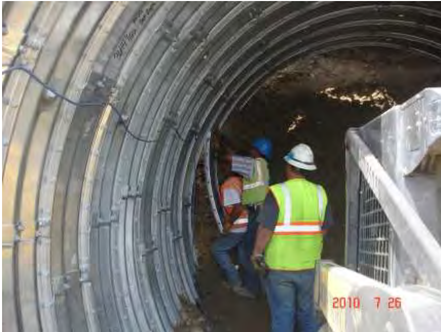
Figure 13: Alkali Creek Tunnel - Liner Plate Assembly
