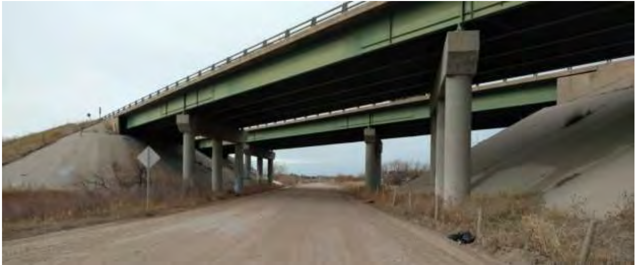
Figure 20: I-80 Bridge over Burlington Trail, Looking Northwest toward Campstool Road
