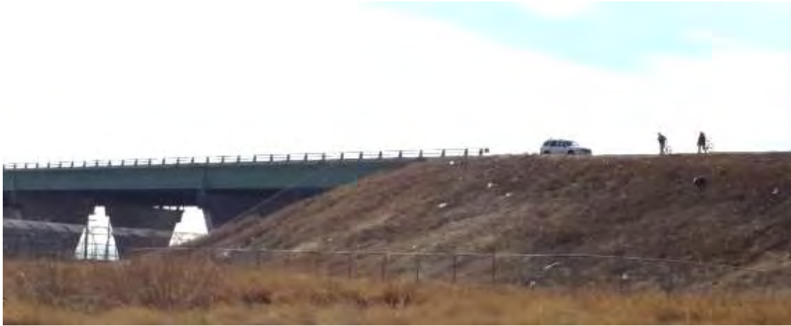
Figure 6: College Drive Bridge over UPRR
