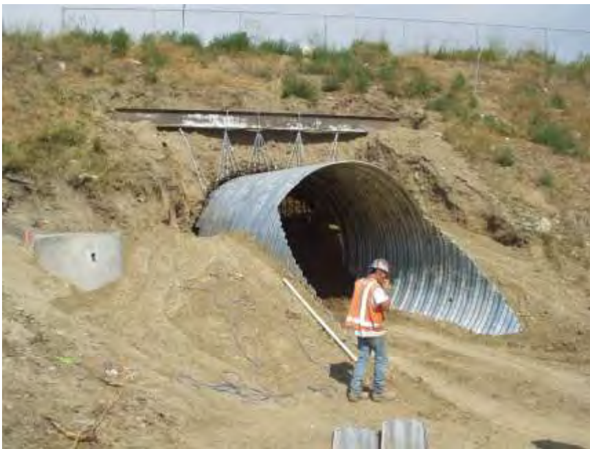
Figure 12: Alkali Creek Tunnel – Excavation to Begin
