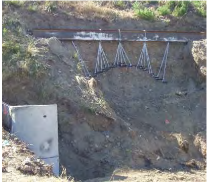
Figure 11: Alkali Creek Tunnel - Earth Support
