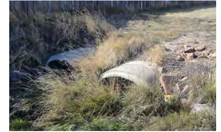
EXISTING CONDITIONS ON CONVERSE AVE.
