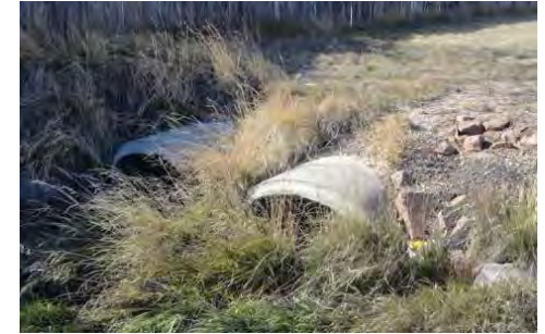
EXISTING CONDITIONS ON CONVERSE AVE.
