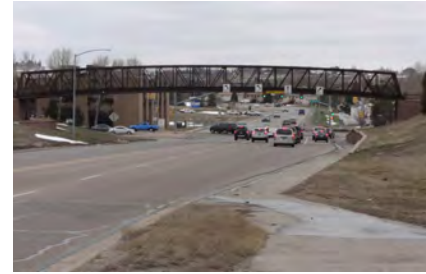
EXISTING PEDESTRIAN BRIDGE ON CONVERSE AVE.
