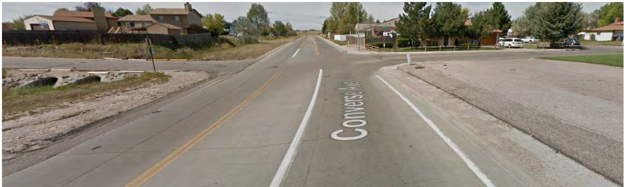
Figure 2. Existing roadway section for Converse Avenue (facing north).
