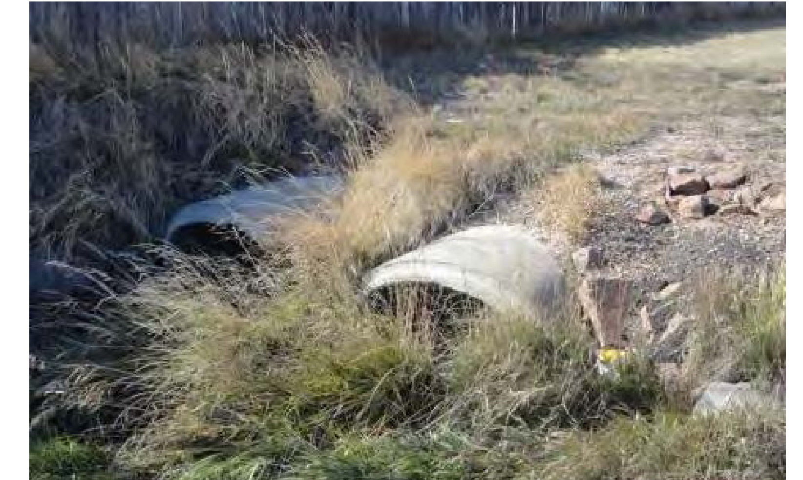
EXISTING CONDITIONS ON CONVERSE AVE.
