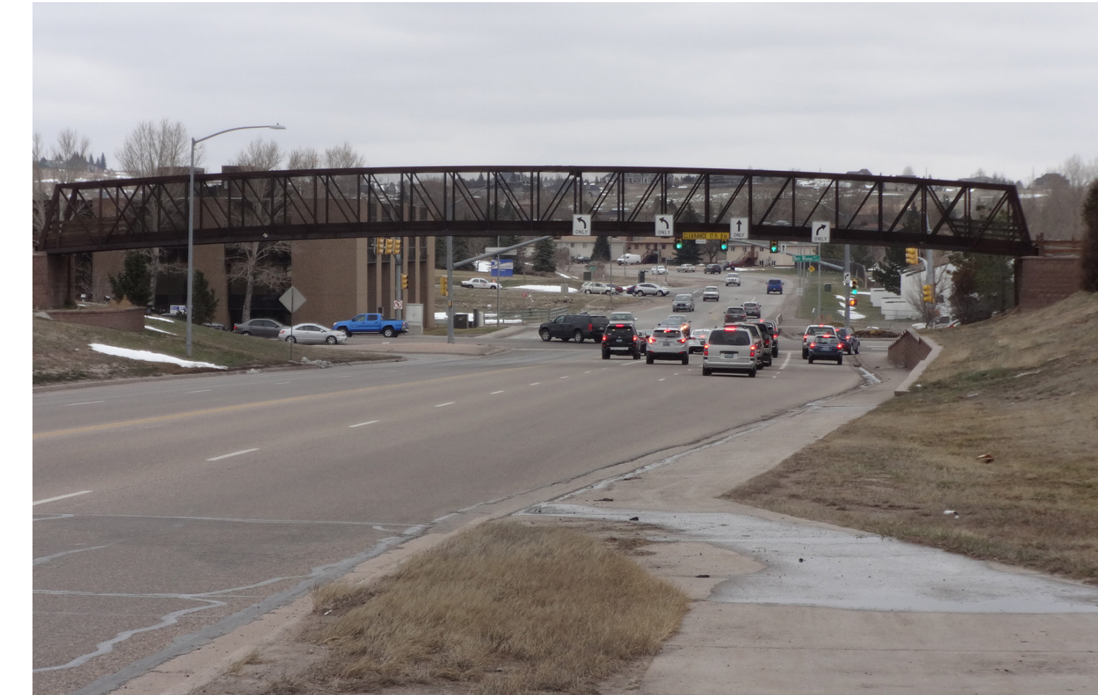
EXISTING PEDESTRIAN BRIDGE ON CONVERSE AVE.
