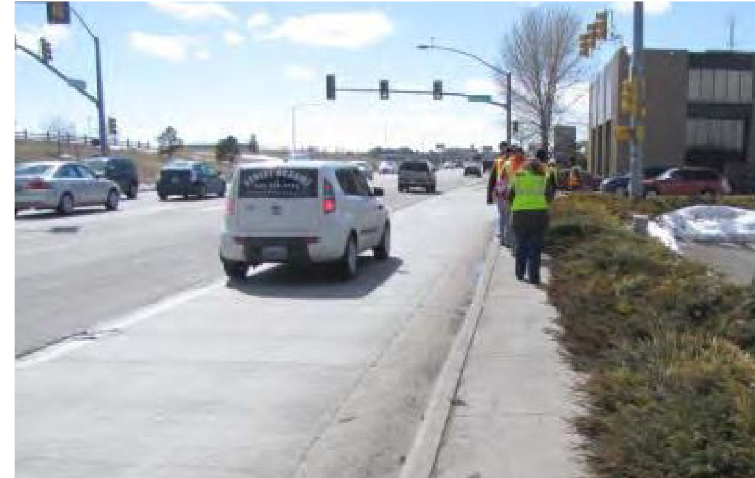
NARROW SIDEWALKS ON DELL RANGE BLVD.
