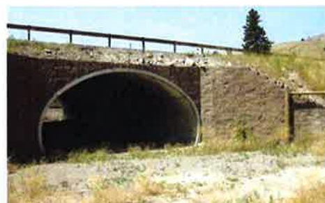
Figure 47. A large-mammal underpass (7-8 m (23-26.2 ft) wide, 4-5 m (13.1-16.4 ft) high) along U.S. Highway 93 south of Ravalli, MT (copyright: Marcel Huijser).
