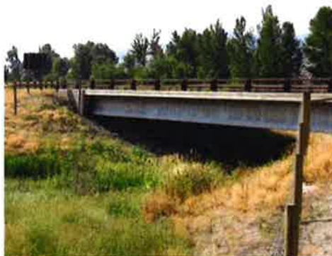
Figure 46. An open-span bridge over Spring Creek, along U.S. Highway 93 south of Ravalli, MT (copyright: Marcel Huijser).
