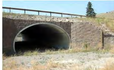
Figure 47. A large-mammal underpass (7-8 m (23-26.2 ft) wide, 4-5 m (13.1-16.4 ft) high) along U.S. Highway 93 south of Ravalli, MT (copyright: Marcel Huijser).
