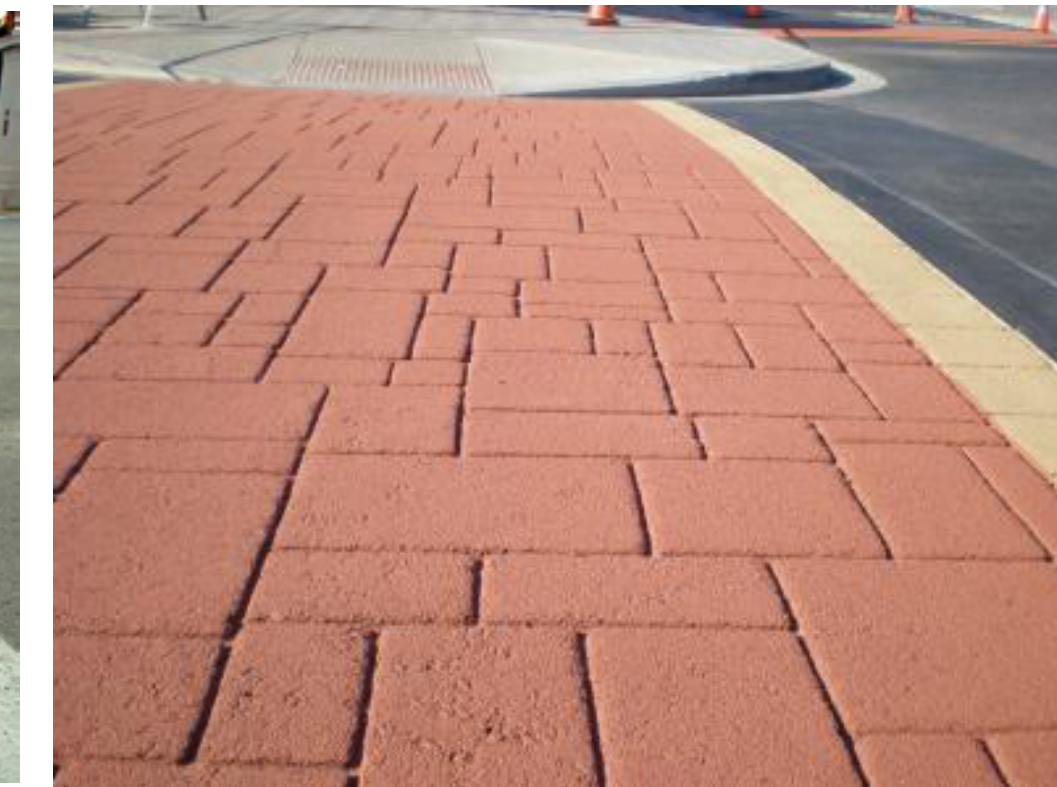
Colored/textured concrete crosswalk
