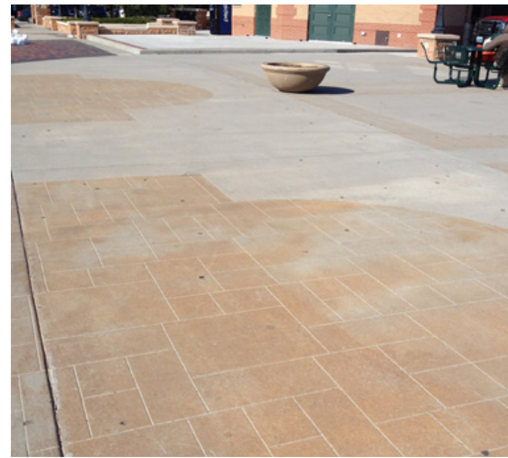
Stained colored concrete
