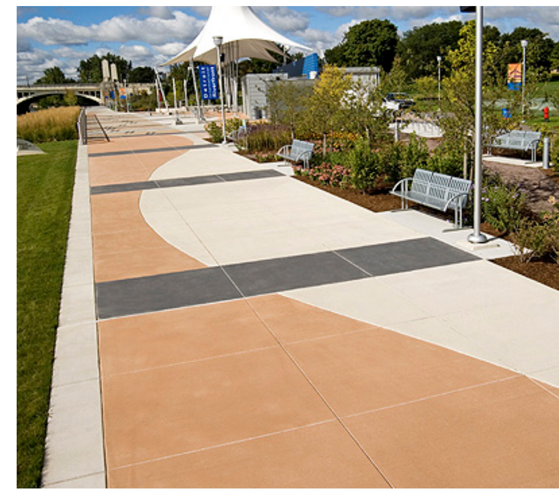
Patterned colored concrete
