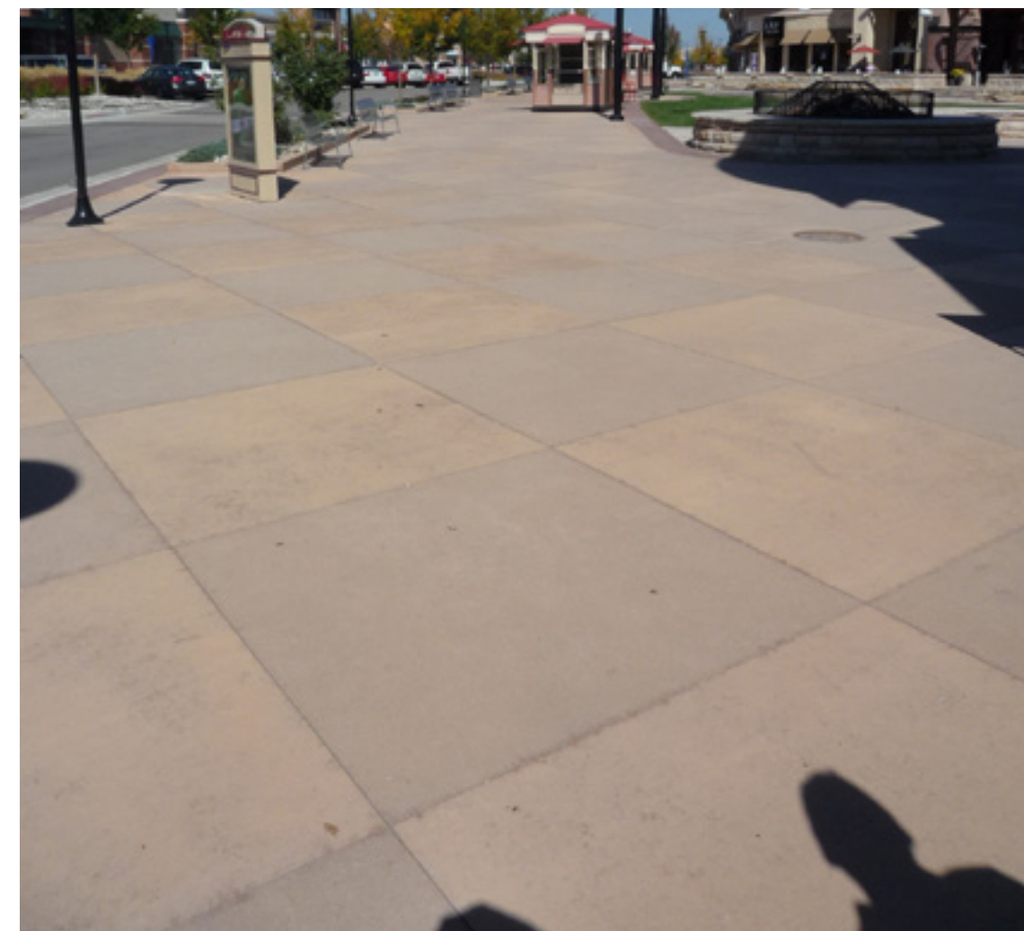
Colored concrete w/sandblasted pattern
