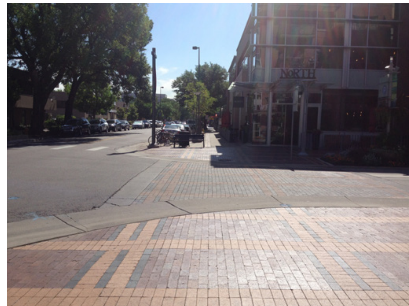
Pavers at intersections
