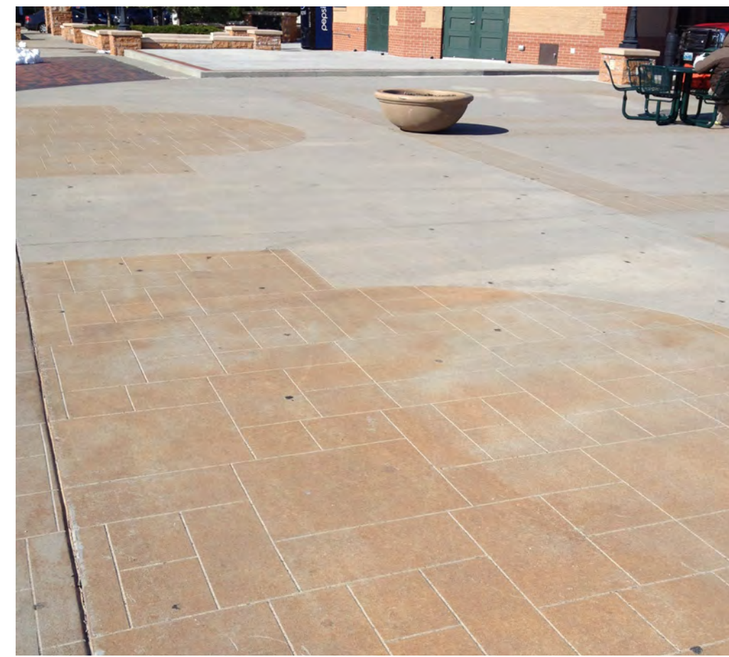
Stained colored concrete
