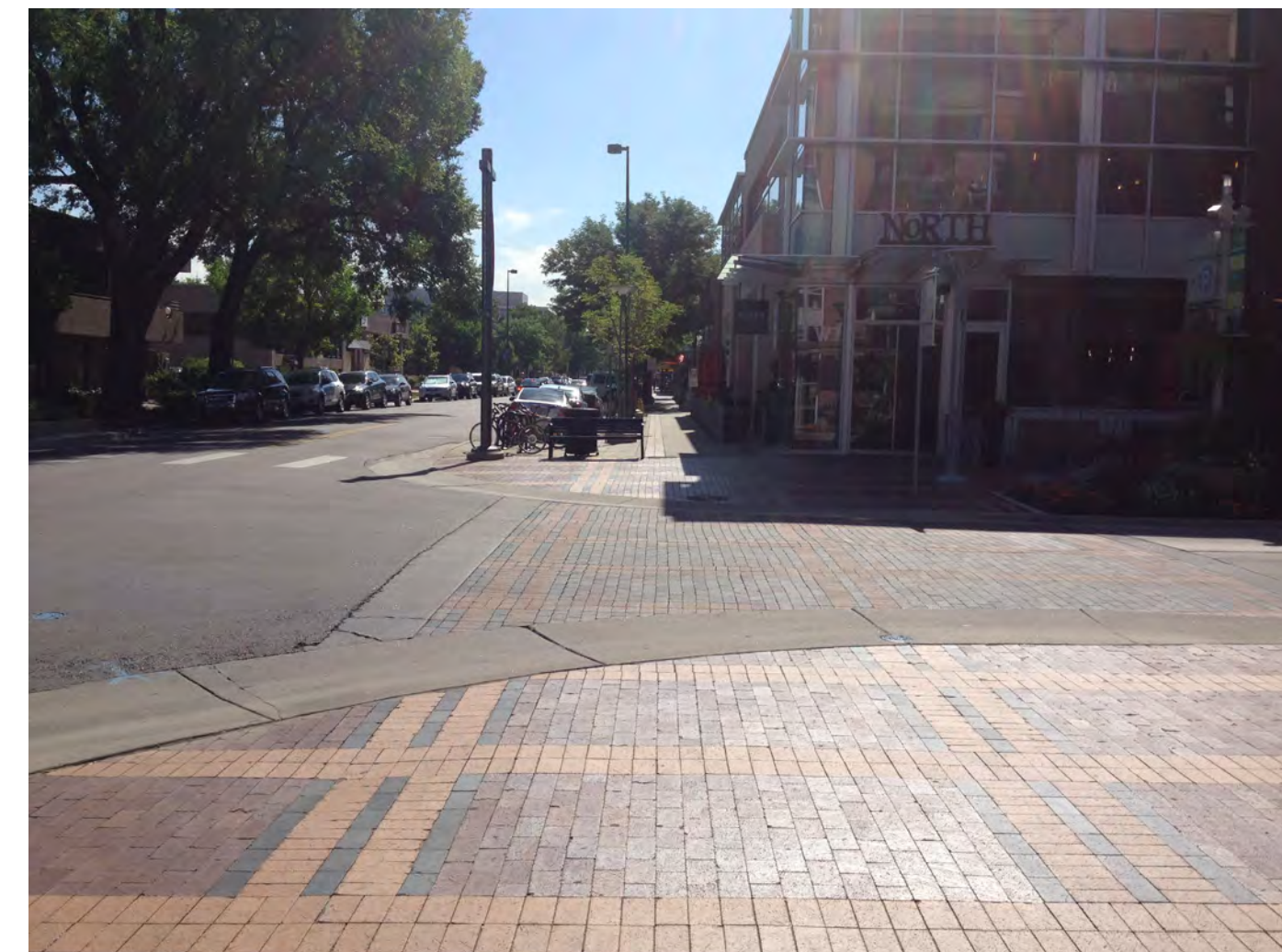
Pavers at intersections
