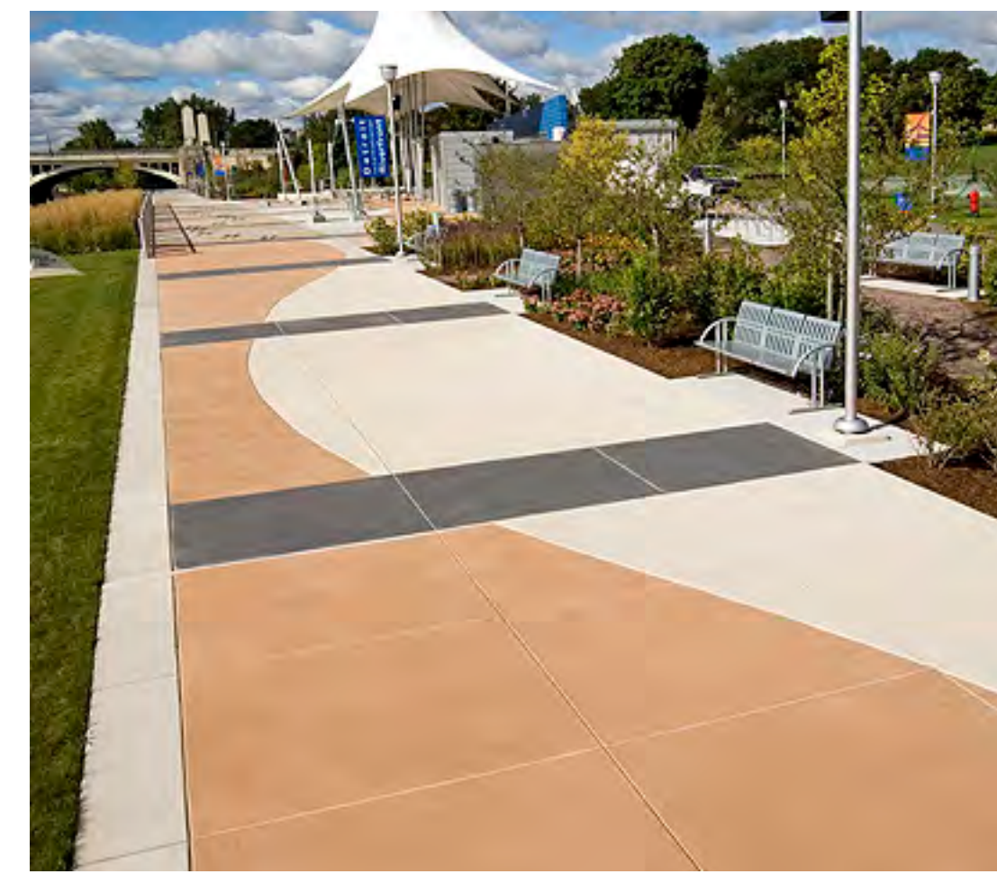
Patterned colored concrete
