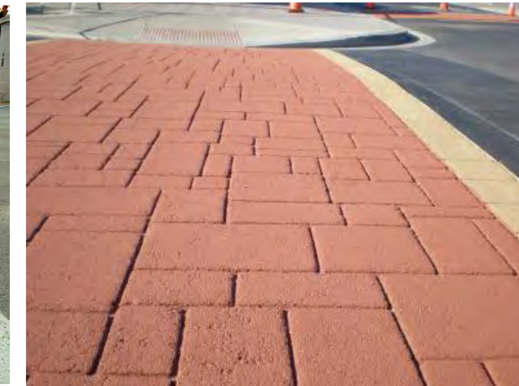
Colored/textured concrete crosswalk
