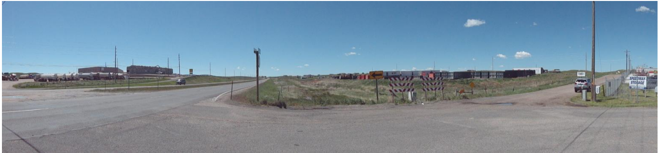
KC Construction and Palomino Industries are at the southeast corner of S. Greeley and High Plains. Stubbs and Stubbs Oilfield Construction Inc. are located on southwest corner and Speedway storage on the northwest corner of this important intersection
