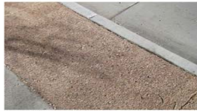
Exposed aggregate crosswalks and retaining walls.
