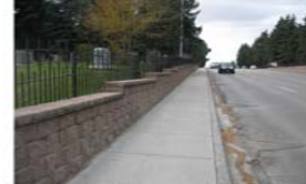
Block Retaining Wall (B1-B2)
