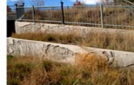
Stamped Concrete Retaining Wall (B3-B4)
