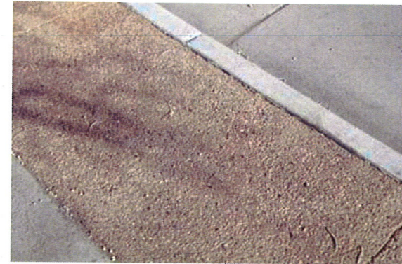
Exposed aggregate crosswalks and retaining walls.
