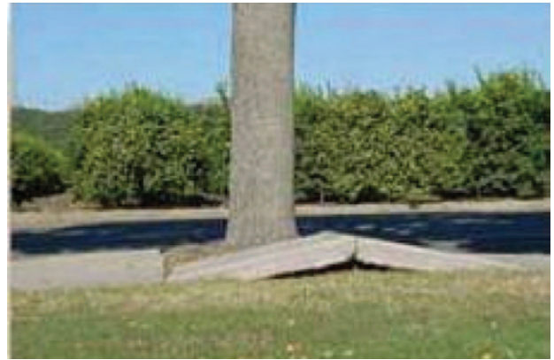
Figure 15. Subsurface tree roots can lift concrete sidewalk slabs, causing the surface to become uneven.
