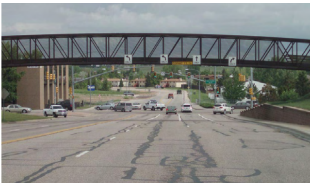
Figure 22. Grade-separated crossings at high-volume roads (such as Converse Avenue) increase pedestrian connectivity and reduce exposure to motor vehicles.
