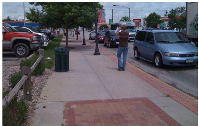
Figure 8. Sidewalks downtown are in good condition and provide sufficient width for several pedestrians to pass each other.
