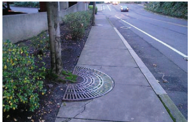
Figure 16. Tree well grates should be flush with the sidewalk surface.
