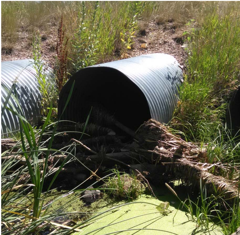
Photo 7.12. Culverts under Education Dr. 3 of 3
