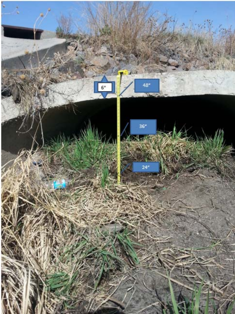
Photo 7.8. Sediment in Culvert No. 3
