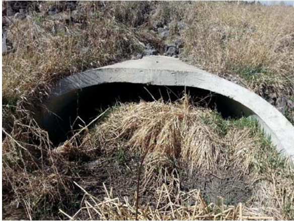
Photo 7.5. Downstream end of Culvert No. 2
