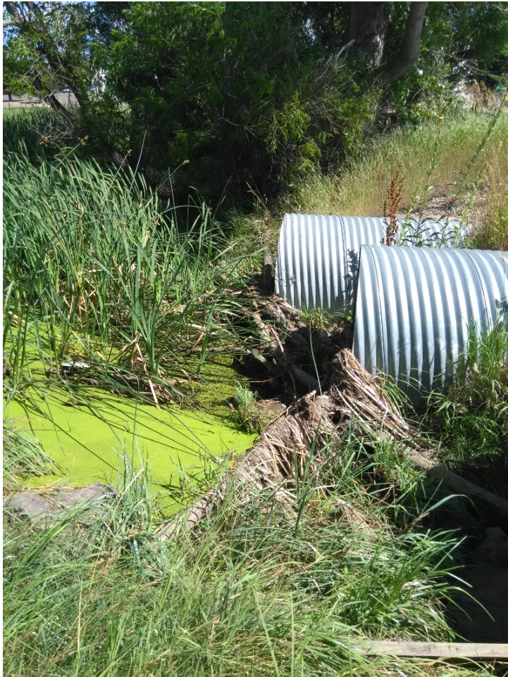
Photo 7.11. Culverts under Education Dr. 2 of 3
