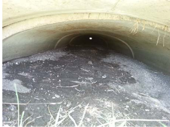
Photo 7.6. Looking Upstream through Culvert No. 2
